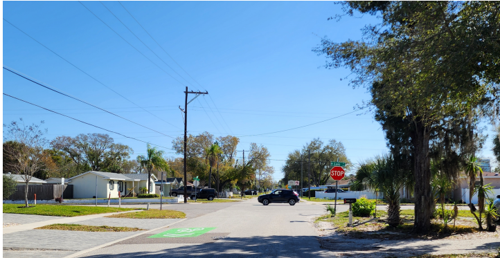
EB View--Approaching Lois Avenue
