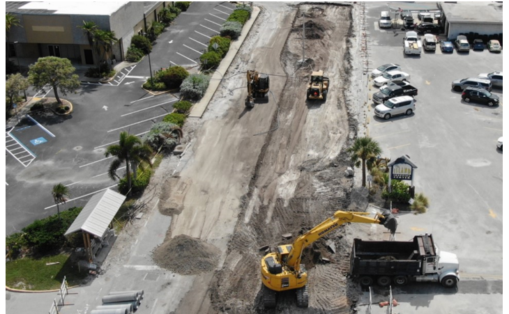
Construction Underway Along Marina Drive
