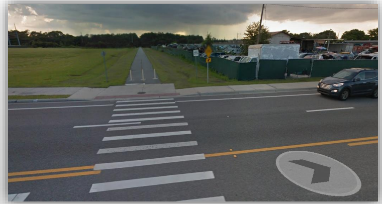
Site qualified for Potential Continuous Bicycle /Pedestrian Counting Shingle Creek Trail, Kissimmee, Florida
