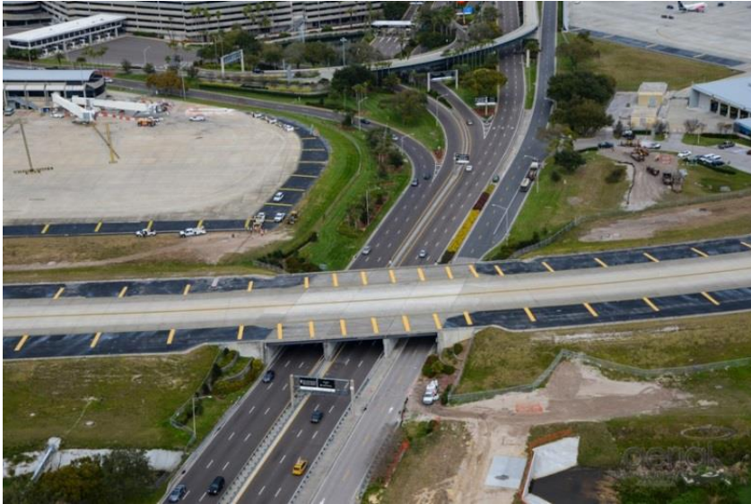
Taxiway J Bridge in February
